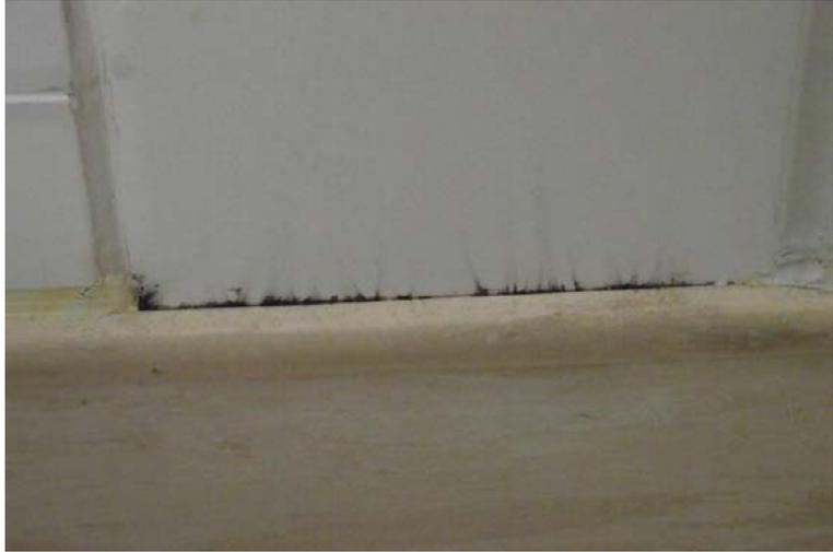
Figure 22. Example of incomplete joints
