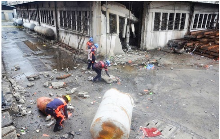
Ice Plant and Cold Storage Building Facility after the ammonia blast incident, Navotas City, Metro Manila, Philippines.
